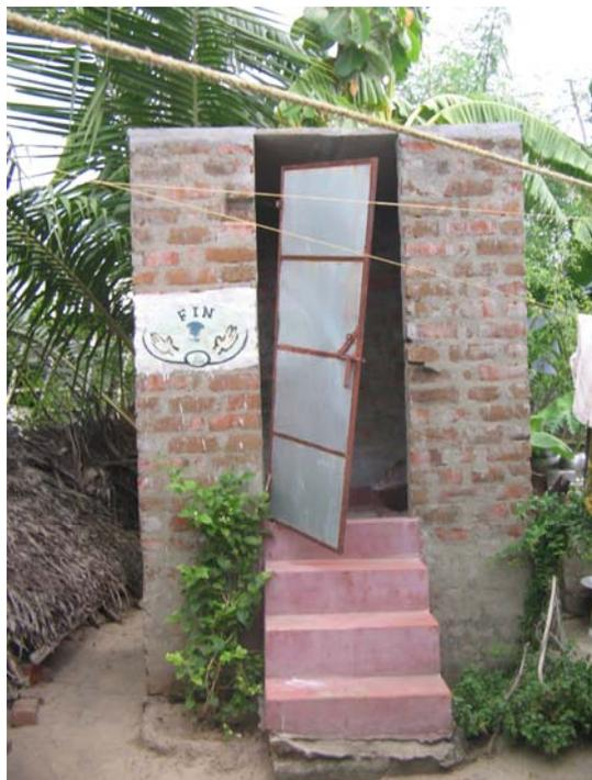
**-Doors that are falling out, falling apart or posing a danger (See left):** The tin sheet used is very inferior. In some cases it is coming out of the doors. The hinges are coming out. Latches are rusty. Latches and bolts for the door are missing. There are a couple of door (4 to 5) which have to be removed each time in order to close the toilet.
